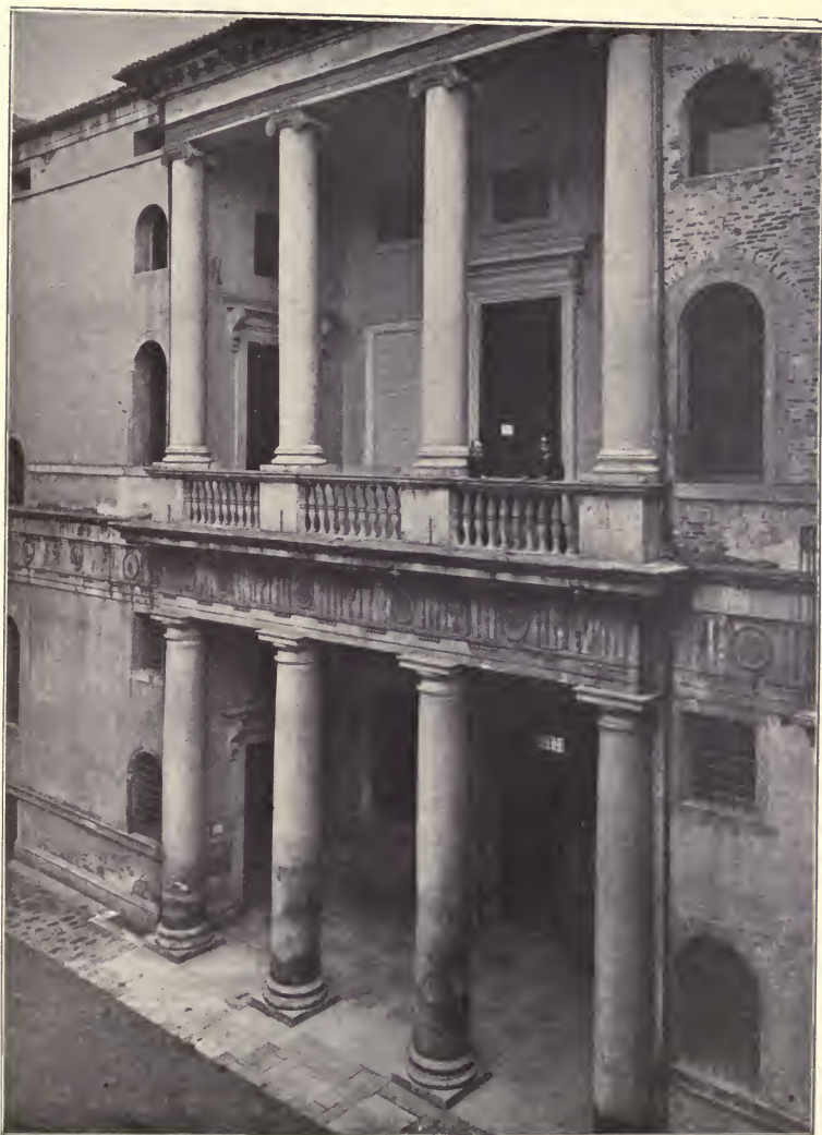
Chiericati Palace, Vicenza, Italy; Andrea Palladio, Architect. Detail of courtyard façade, showing Renaissance use of Ionic over Doric Order, both being of exceptionally refined and Classic proportions. (Compare with detail of Theater of Marcellus opposite page 198.)
