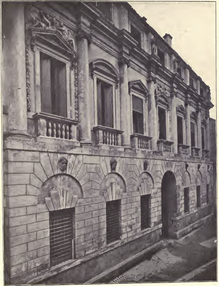
Colleoni-Porto Palace, Vicenza, Italy; Andrea Palladio, Architect. A Renaissance example of the placing of an Order above an arcade.
