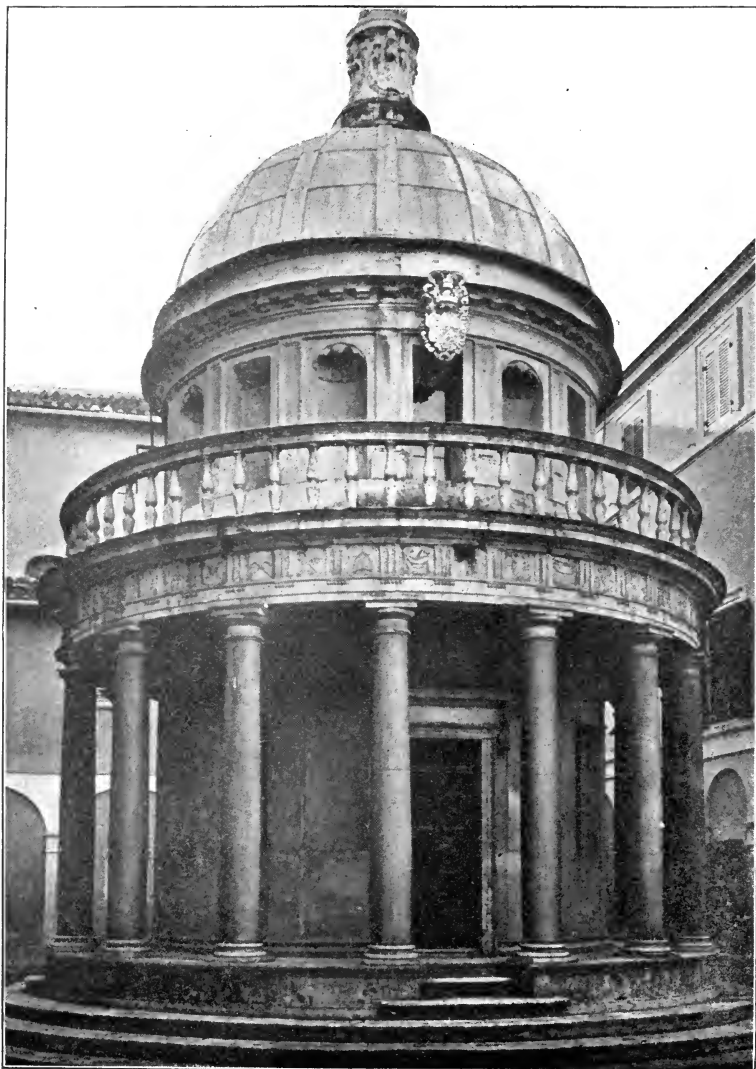
Circular Temple In Courtyard of San Pietro, Montorio, Rome; Donato d'Angnolo Bramante, Architect Showing Renaissance use of Doric Order in a circular temple with domed lantern above.
