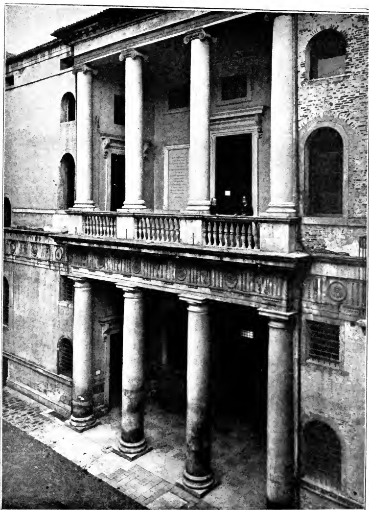
Chiaregati Palace, Vicenza, Italy; Andrea Palladio, Architect. Detail of courtyard façade, showing Renaissance use of Ionic over Doric Order, both being of exceptionally refined and Classic proportions. (Compare with detail of Theater of Marcellus opposite page 138.)
