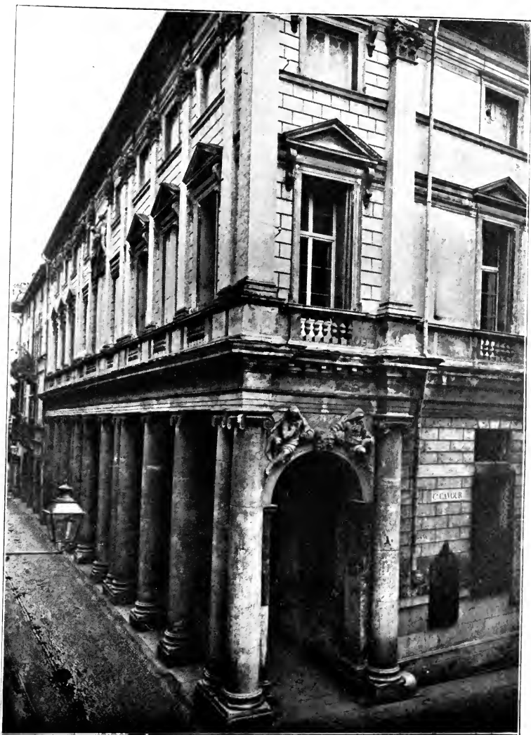
Porto Palace, Vicenza, Italy (1588); Vincenzo Scamozzi, Architect. A Renaissance example of the use of Composite pilasters over an Ionic colonnade.
