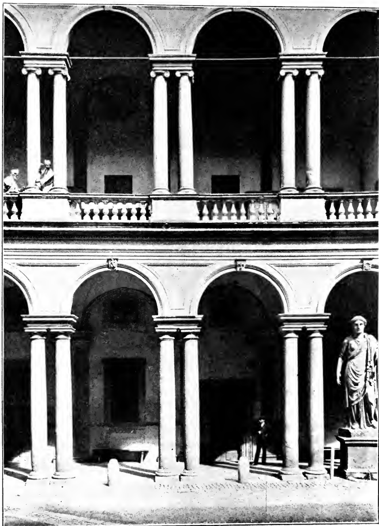
Detail of Courtyard, Borgnese Palace, Rome; Martino Longhi, Architect. Showing Renaissance superposition of arches resting on coupled columns.
