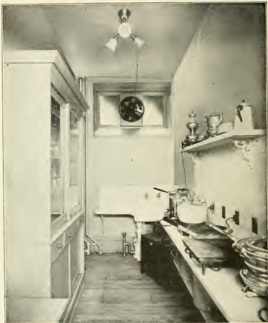
ELECTRICAL KITCHEN IN EDISON BUILDING, CHICAGO
