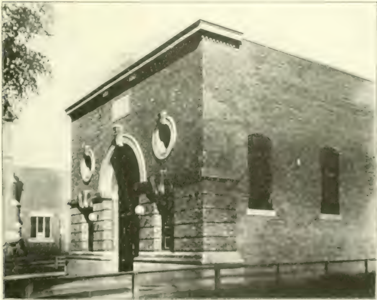
Ohio Street Substation.
