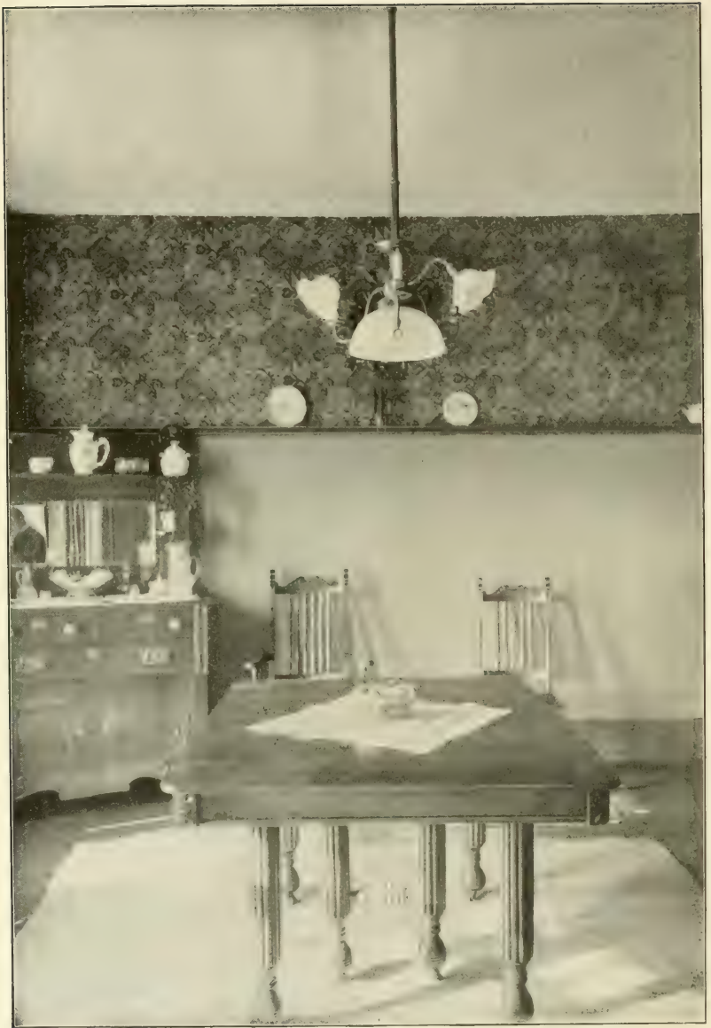
SIMPLE COMBINATION GAS AND ELECTRIC FIXTURE IN A DINING ROOM
