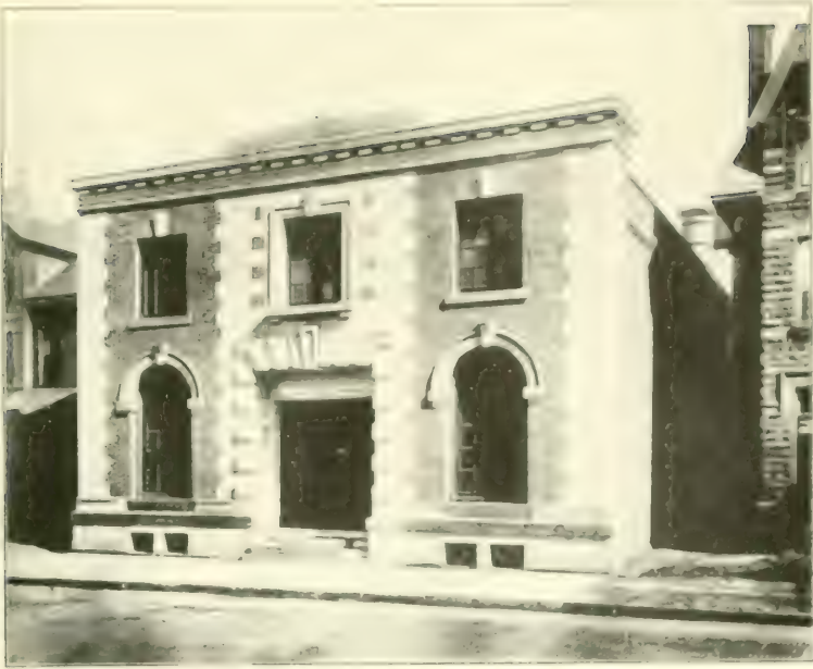
Dodge Street Substation.
