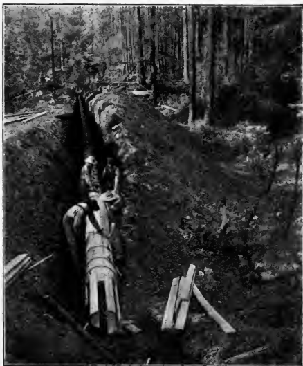
Fig. 15. Erecting a 12-Inch Pipe of California Redwood.
