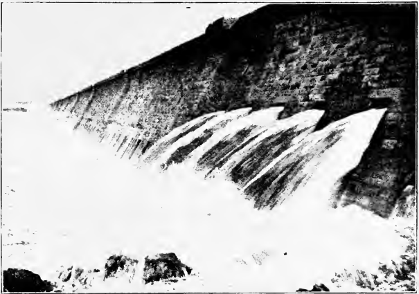
Fig. 9. Assuan Dam, River Nile, Egypt.
