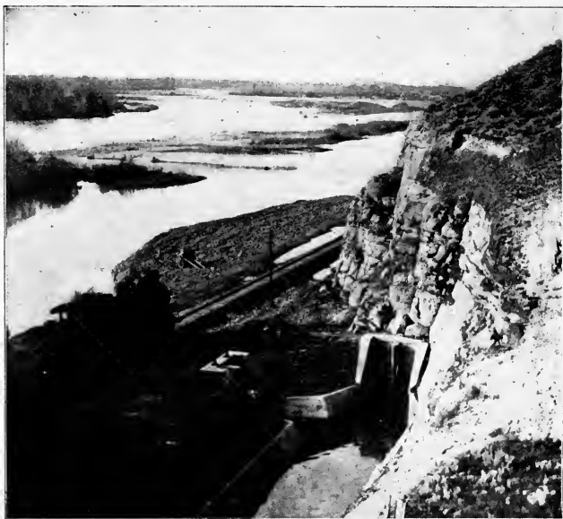
Fig. 14. General View of Wasteway and Portal of Tunnel No. 3 on Huntley Main Canal, and Passing Northern Pacific Train.
