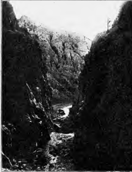
Fig. 22. Government Dam Site, Shoshone River, Wyoming. Reservoir to store 300,000 acre-feet. Height of dam to be 210 feet; walls of canyon 700 feet high. Diamond drills bored 80 feet below river bed before striking solid foundation rock.
