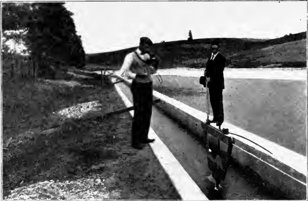
Fig. 28. U. S. Geological Survey Rating Station at Los Angeles, California. Here the meters used in the measurement of the flow of streams are calibrated.
