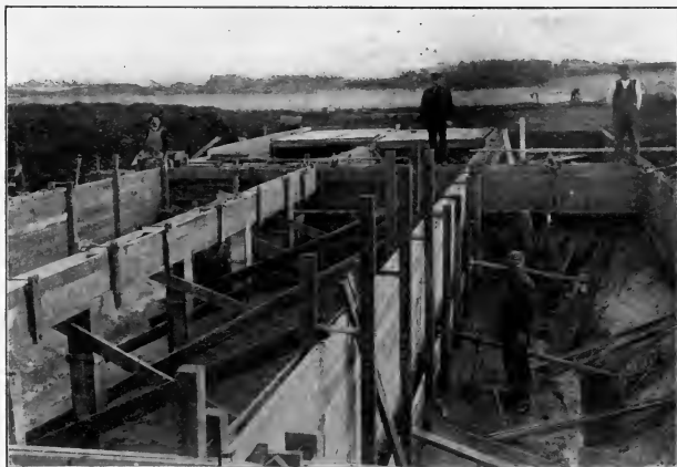
Fig. 45. Septic Tank at Carroll, Iowa, under Construction.
