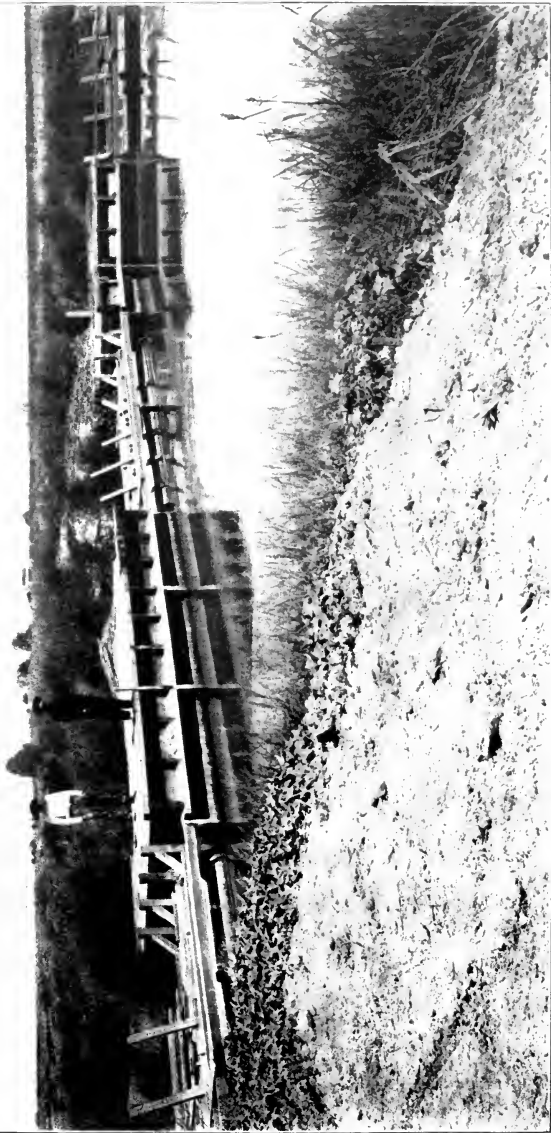
HEADINGS CONTROLLING SUPPLY OF WATER FOR THE SMALLER LATERALS FROM THE MAIN IMPERIAL CANAL
