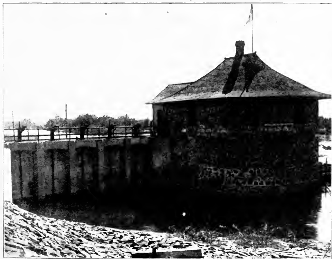
Fig. 7. Gate House and Intake Gates, Upstream Face, Sunnyside Canal.
