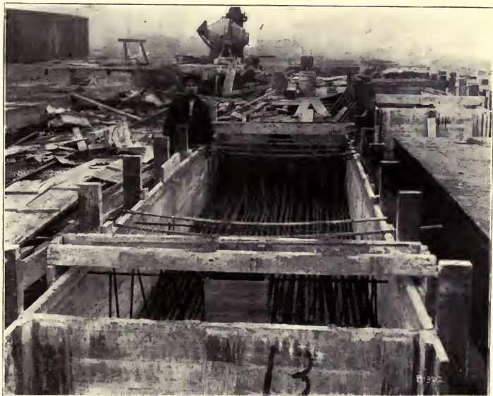
Form Box, with Reinforcing Bars, for Construction of Slabs Shown Above.
