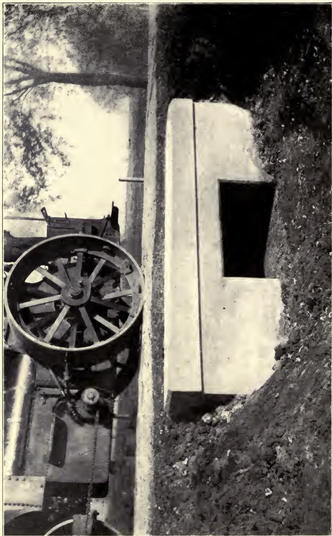
ROAD ROLLER TESTING A CONCRETE CULVERT
