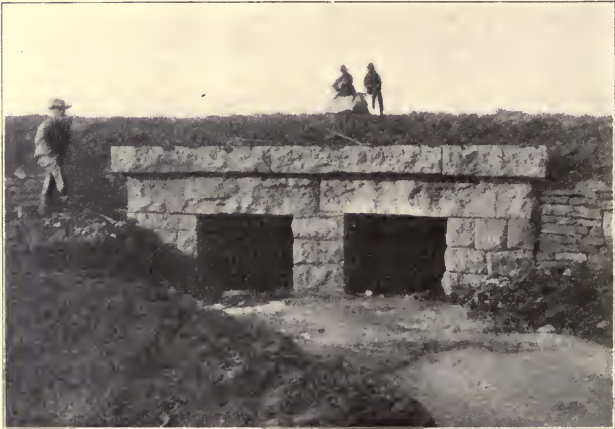
Fig. 75. Double Box Culvert, 4 by 3-Foot.
