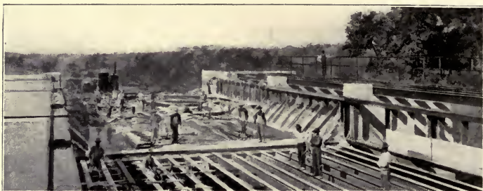
Depositing Concrete for Lining of Aqueduct No. 7.
