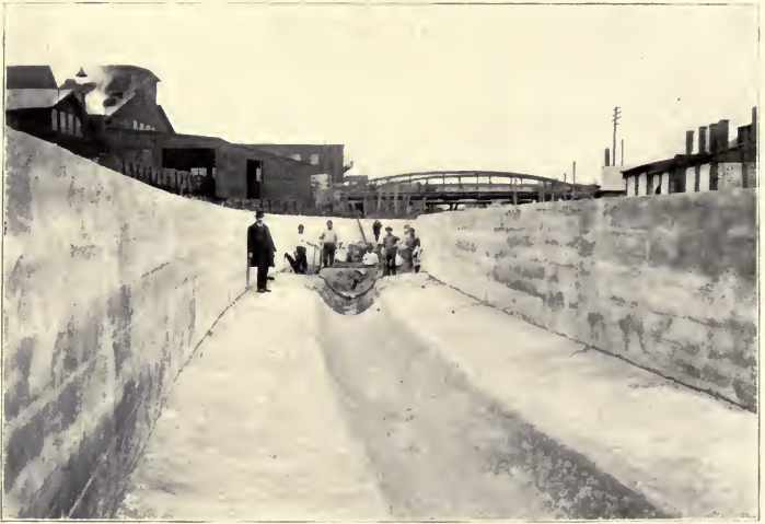
Large Concrete Sewer in Aramingo Canal.
