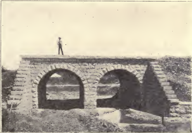
Fig. 77. Double Arch Culvert, 14 by 5½-Foot.
