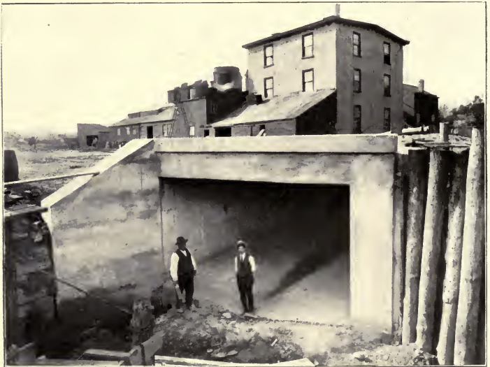
Wakeling Street Concrete Sewer, 16 ft. by 10 ft. 6 in.
