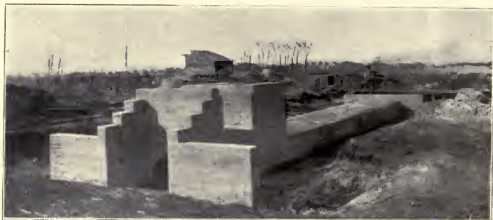
Reinforced-Concrete Arch Culvert, Completed.
