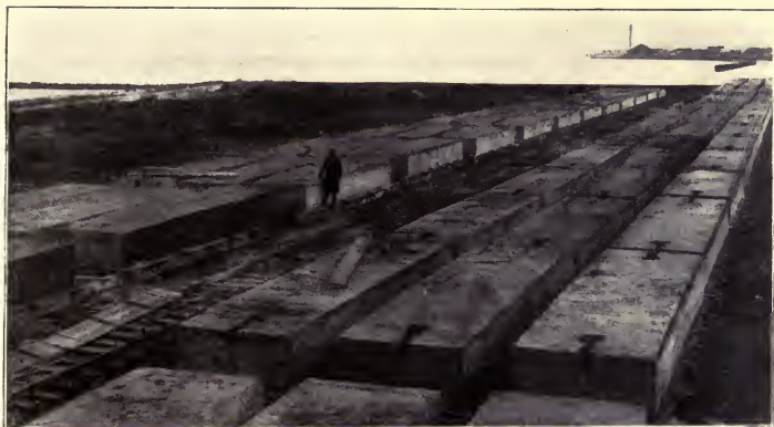
Reinforced-Concrete Bridge Slabs in Storage Yard of Illinois Central Railway, Chicago.
