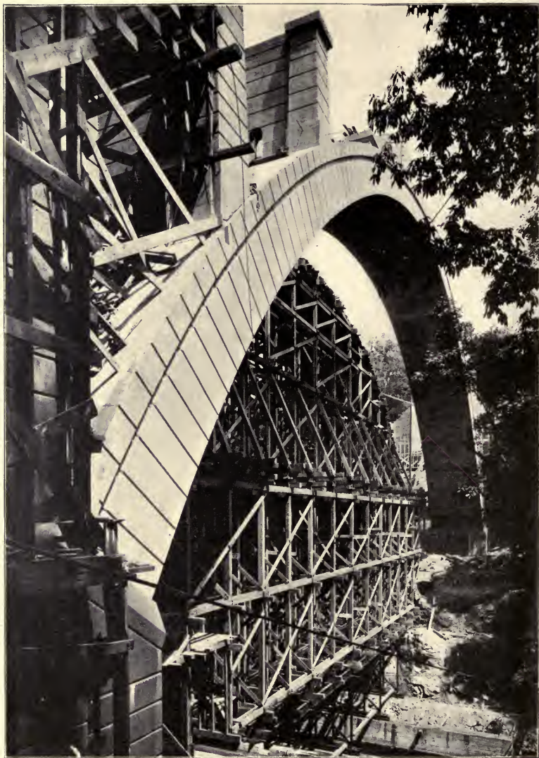
REINFORCED-CONCRETE ARCH RIB, WALNUT LANE BRIDGE, PHILADELPHIA, PA.
