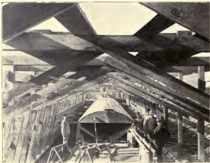
Forms for Construction of Arched Culvert Shown Above.
