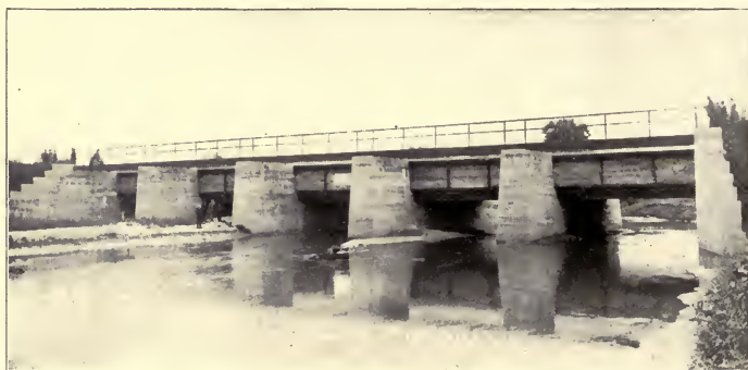
View of Completed Aqueduct.
