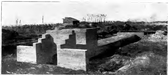
Reinforced-Concrete Arch Culvert, Completed.
