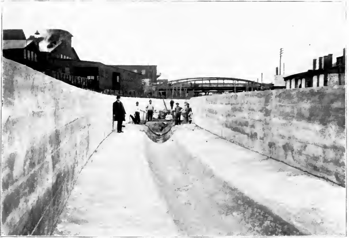
Large Concrete Sewer in Aramingo Canal.
