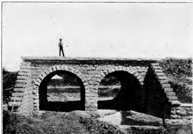
Fig. 77. Double Arch Culvert, 14 by 5½-Foot.
