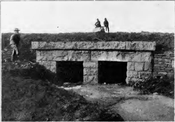
Fig. 75. Double Box Culvert, 4 by 3-Foot.
