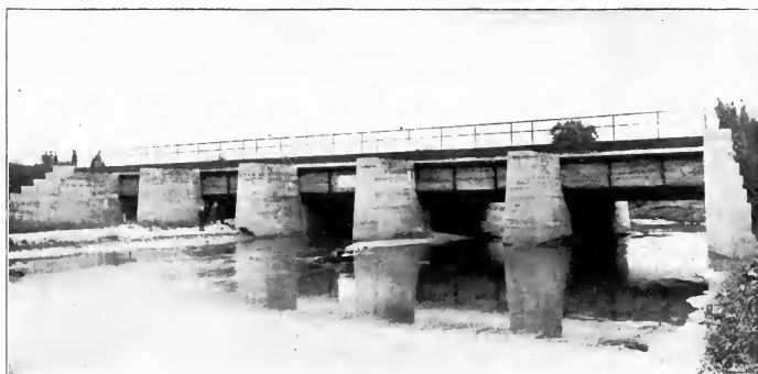
View of Completed Aqueduct.
