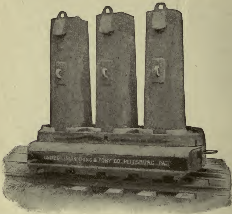
Fig. 11. Steel Ingots Incased in the Molds and Resting on Car From Stoughton's Metallurgy of Iron and Steel Courtesy McGraw-Hill Publishing Company
