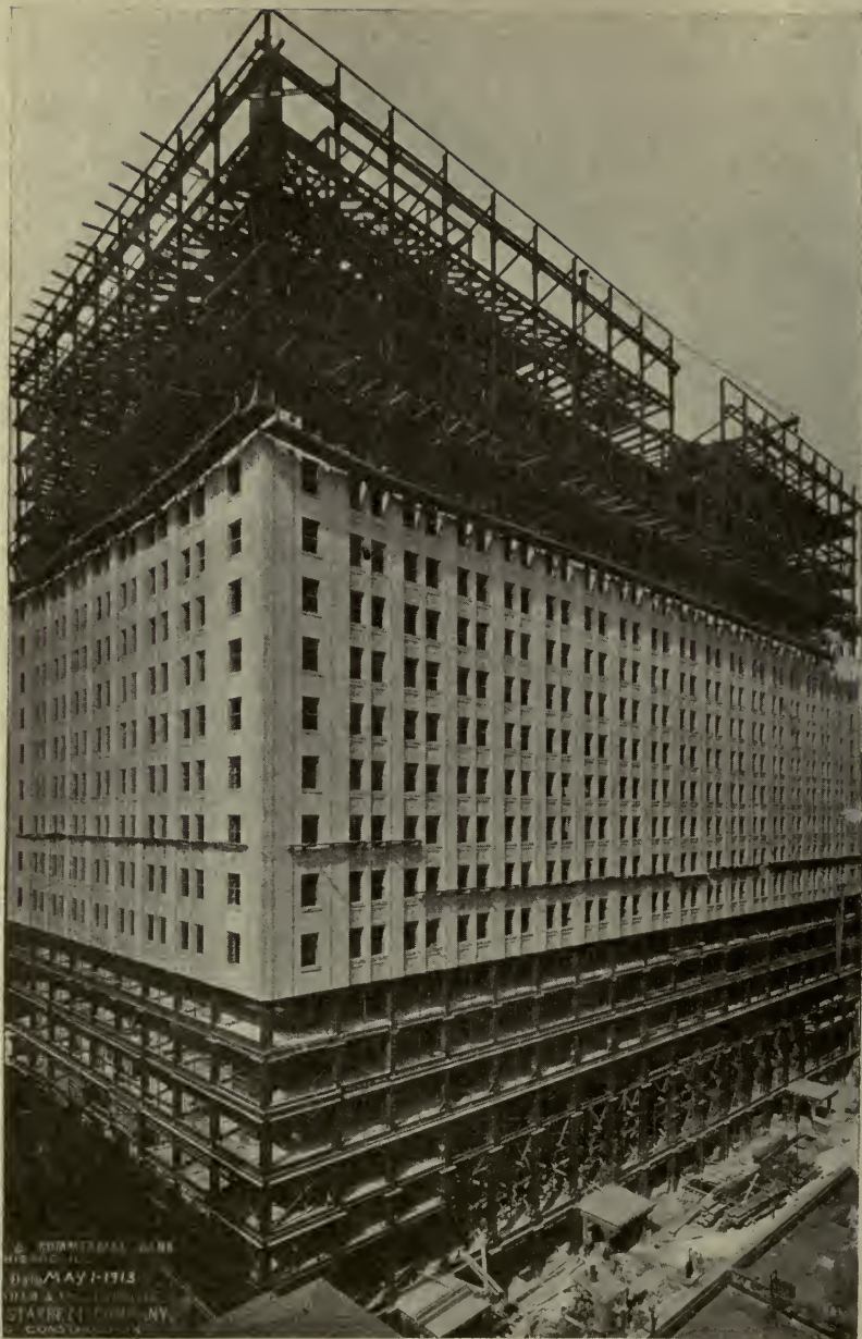
CONTINENTAL AND COMMERCIAL BANK BUILDING, CHICAGO, IN PROCESS OF CONSTRUCTION
