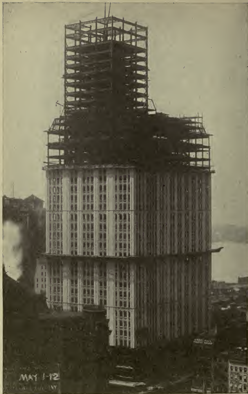
WOOLWORTH BUILDING IN PROCESS OF CONSTRUCTION Cass Gilbert, Architect
