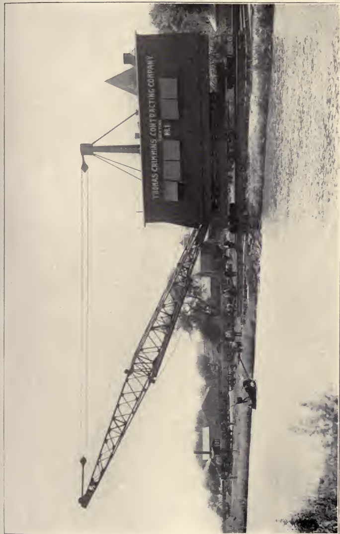
LIDGERWOOD-CRAWFORD SCRAPER BUCKET EXCAVATOR Courtesy of Lidgerwood Manufacturing Company, New York City
