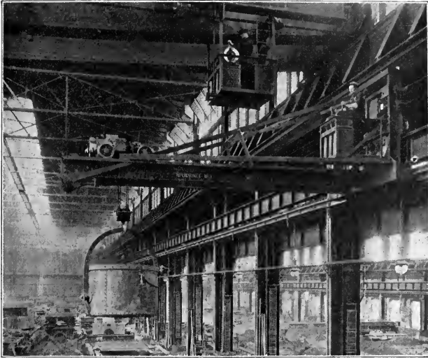
Fig. 109. Wall Jib-Crane, Electrically Operated; Capacity, 10,000 Lbs. Courtesy of Pawling & Harnischfeger, Milwaukee, Wisconsin.
