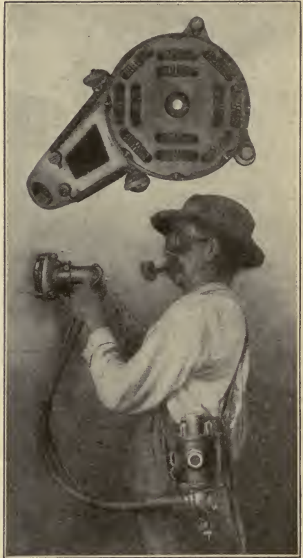
Fig. 196. Power-Driven Hand Tool for Surfacing Concrete
