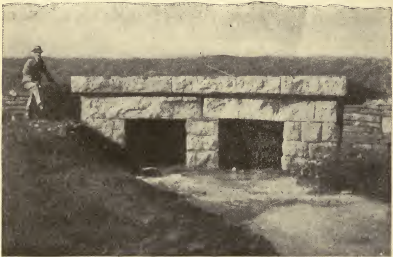
Fig. 74. Double Box Culvert. Openings 4 by 3 Feet
