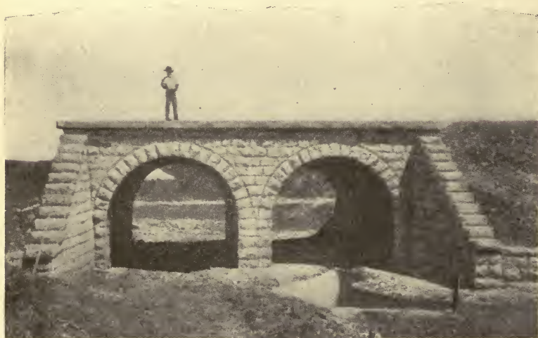
Fig. 76. Double Arch Culvert. Openings, 14 by 5½ Feet
