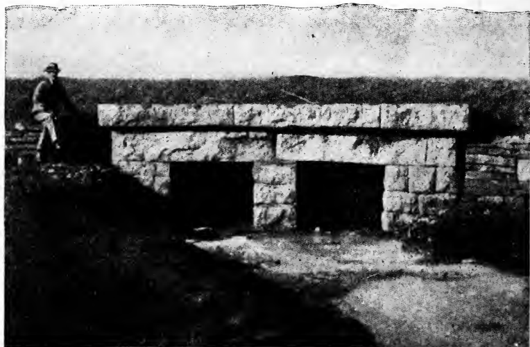
Fig. 74. Double Box Culvert. Openings 4 by 3 Feet
