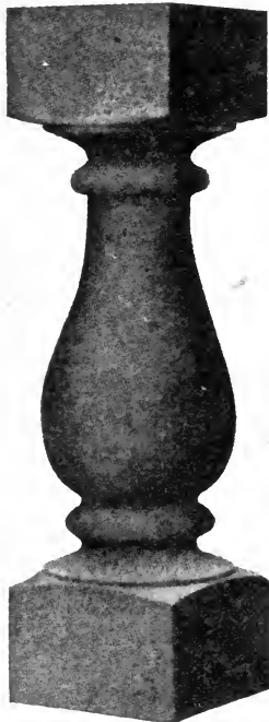
Fig. 198. Typical Molded Concrete Baluster
