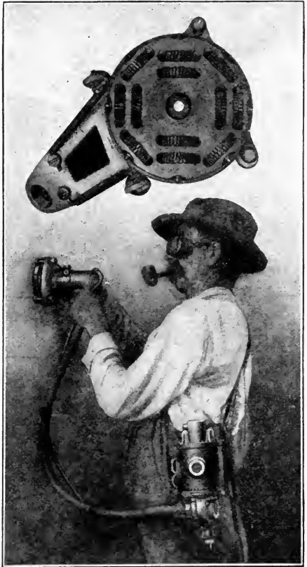
Fig. 196. Power-Driven Hand Tool for Surfacing Concrete
