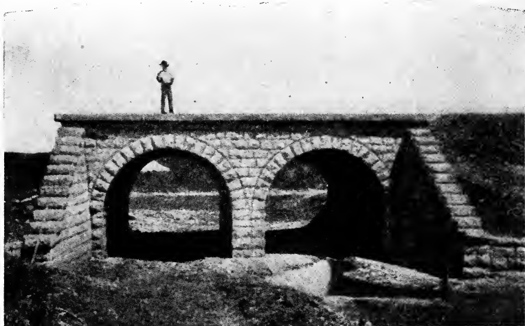
Fig. 76. Double Arch Culvert. Openings, 14 by 5½ Feet
