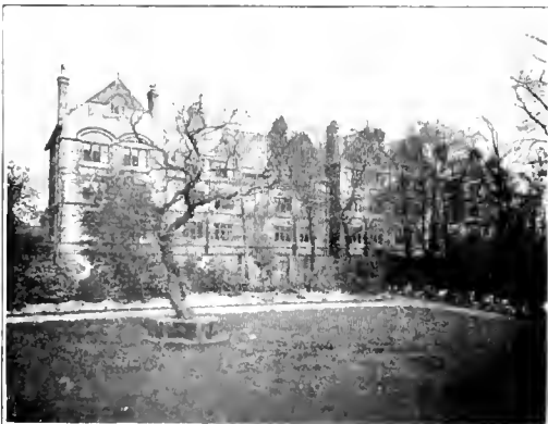
Dalton Hall, Manchester University A Modern City Dormitory.
