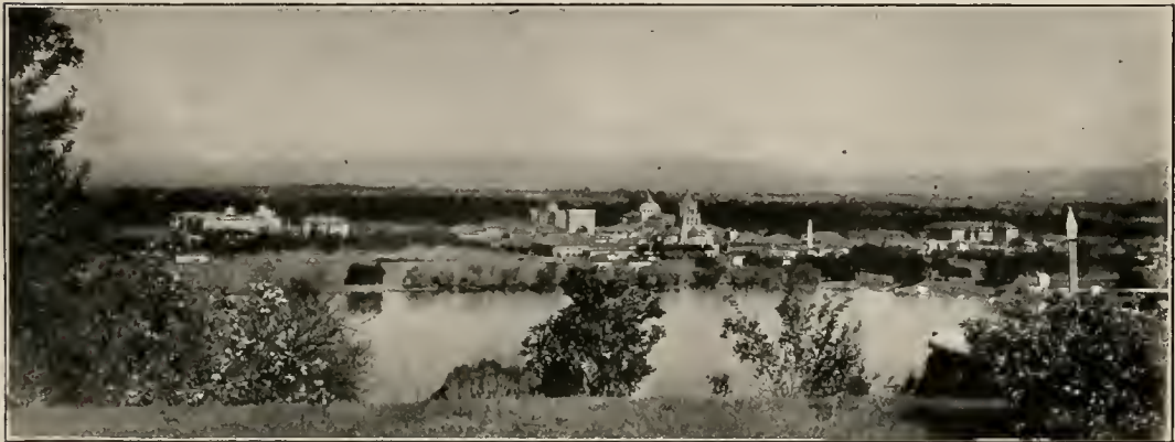
Bird's-eye View from Foothills to the Rear.
