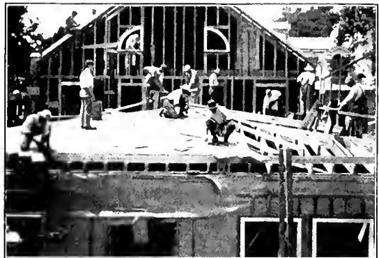
Instruction in Carpentering.
