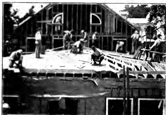
Instruction in Carpentering.
