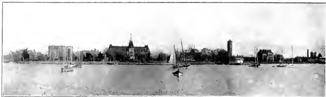
General View from Hampton Roads.
