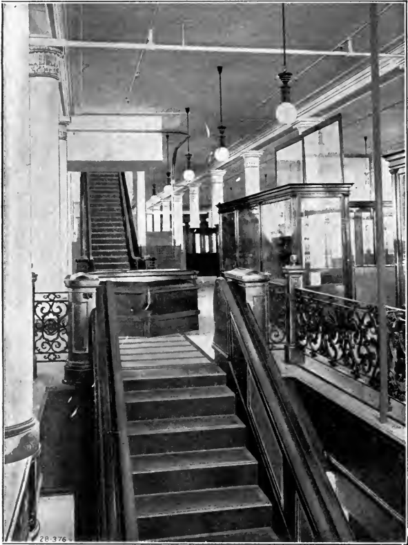
ESCALATORS IN A CITY STORE.
