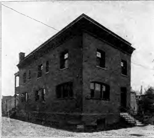
Fig. 22. Modern Light and Power Substation.
