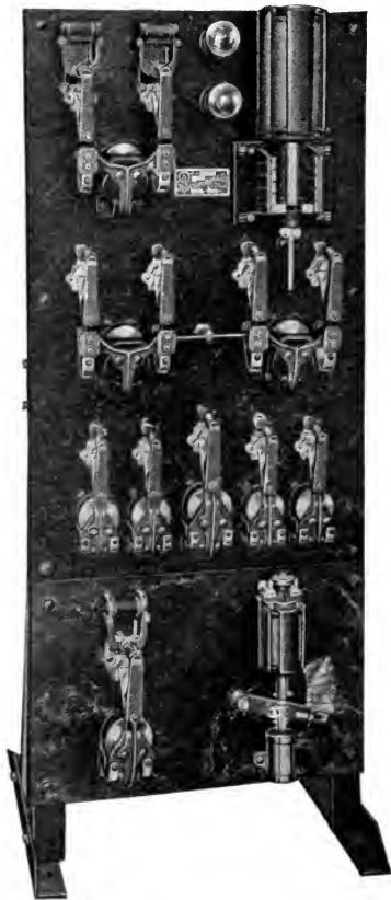
Fig. 19. Electrically Operated Controller.
