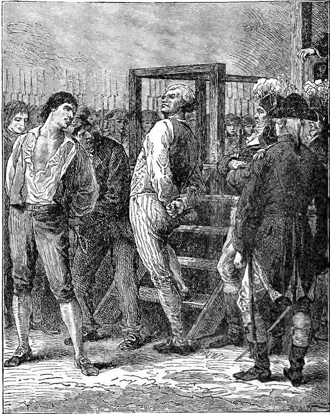
DANTON MOUNTING THE SCAFFOLD.
