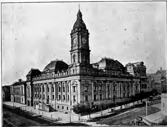
TOWN HALL, MELBOURNE, AUSTRALIA.
