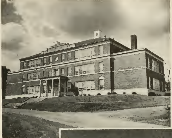
The Science Building
