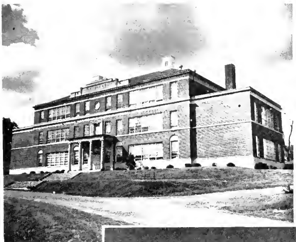
The Science Building
