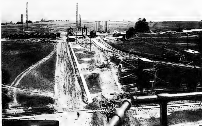
Construction of Main Battery at the Lower Station.
