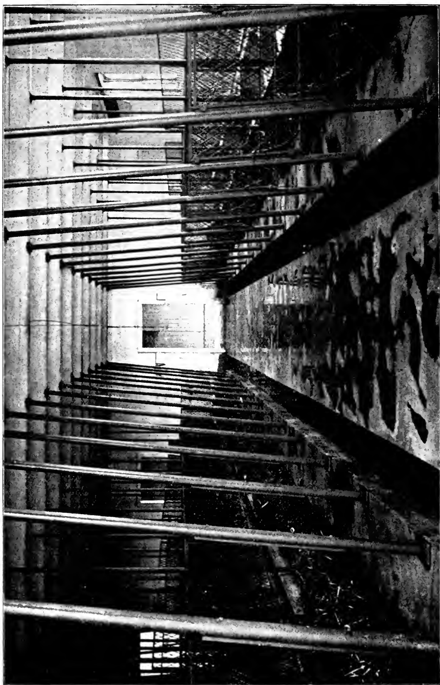
CUT 43. A SANITARY DAIRY BARN FOR THE PRODUCTION OF CERTIFIED MILK. CEMENT FLOOR, IRON STALLS, SIDES WHITEWASHED, WELL LIGHTED AND PROVIDED WITH A GOOD SYSTEM OF VENTILATION. EXTERIOR SHOWN IN CUT 12.
