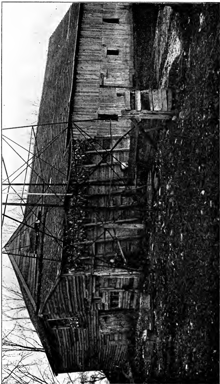
CUT 13. PORTION OF BARN ON RIGHT IS A STABLE FOR 36 COWS. NO PROVISION FOR LIGHT OR VENTILATION; OPENINGS SHOWN ARE COVERED WITH BOARDS IN WINTER. MUD HOLE IN YARD; MARKS ON BARN SHOW WHERE MANURE HAS BEEN PILED.
