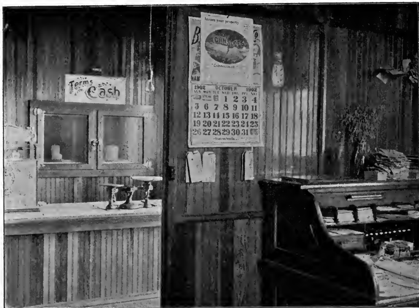
CUT 26. OFFICE. DOOR OPEN INTO ENTRANCE, SHOWING COUNTER, AND GLASS DOORS IN REFRIGERATOR.
