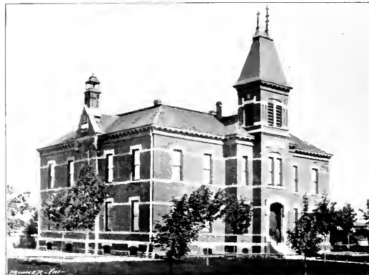
VALE SCHOOL BUILDING.
