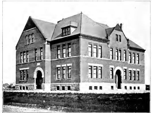
BAXTER SCHOOL BUILDING.
