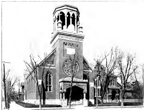
ST. PAUL'S PROTESTANT EPISCOPAL CHURCH. Built 1846. Rebuilt 1892.
