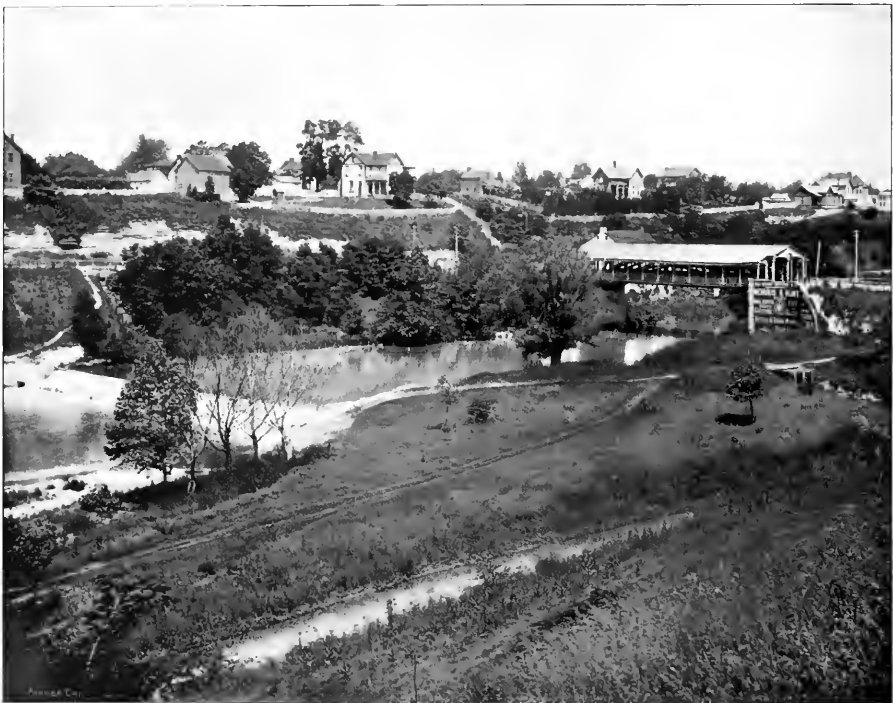
VIEW ON WHITE WATER RIVER, SHOWING OLD NATIONAL BRIDGE.
