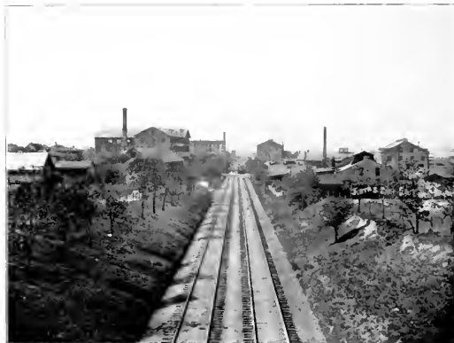
VIEW OF RAILROAD, LOOKING WEST FROM NINETEENTH STREET BRIDGE.
