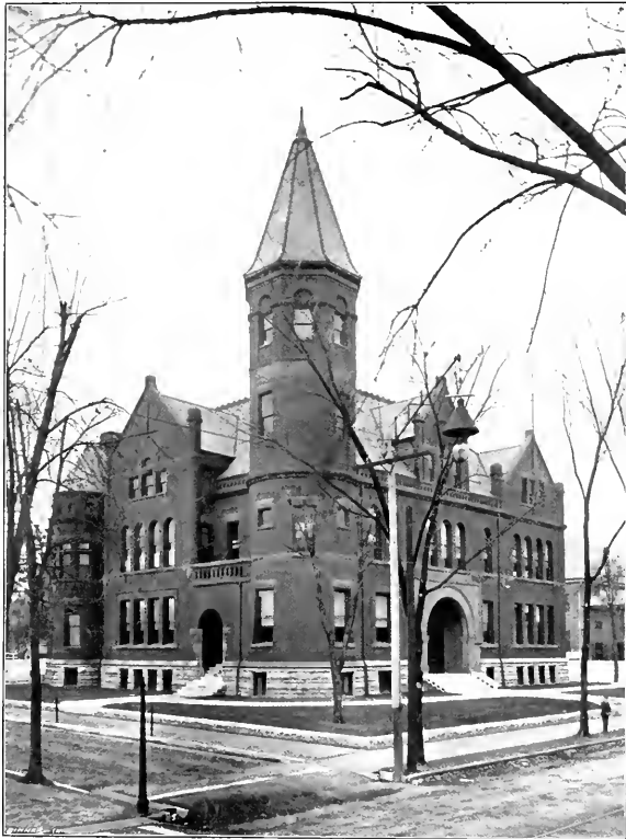
GARFIELD SCHOOL BUILDING.
