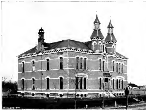
WHITWATER SCHOOL BUILDING.
