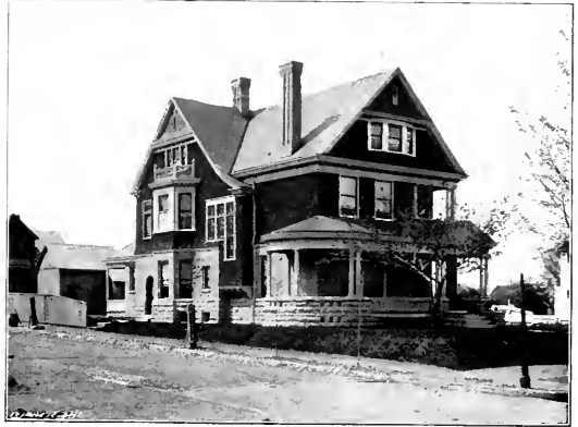
RESIDENCE OF JOHN A. HASEGOSTER, ARCHITECT, S. W. COR 20TH AND MAIN STS.
