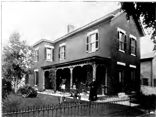
RESIDENCE OF H. H. MEERHOFF.
