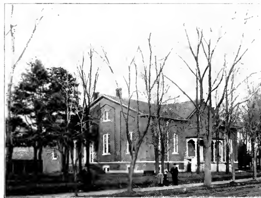
INDIANA YEARLY MEETING HOUSE, (HICKSITE.) ERECTED 1905.
