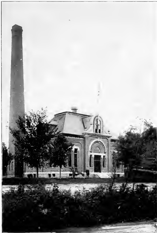
RICHMOND CITY WATER WORKS.
