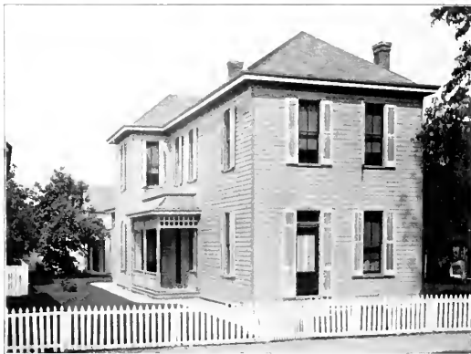
RESIDENCE OF JOHN H. MEERHOFF.
