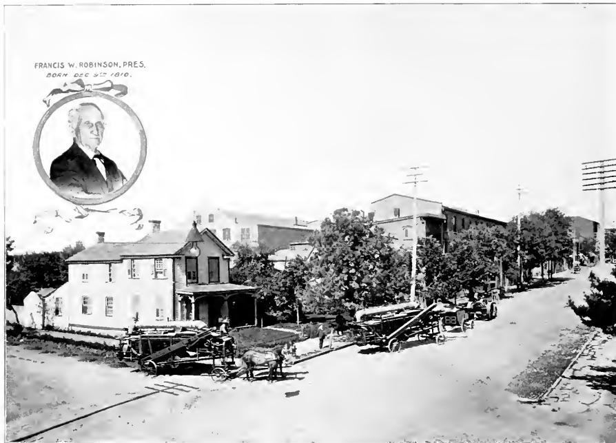
OFFICE AND MAIN STREET FRONT OF ROBINSON MACHINE WORKS.
