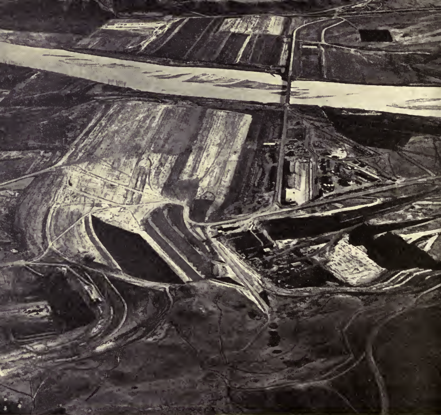
10. Garrison Dam on the Missouri River, North Dakota. Outlet works will go under the curving portion of the dam in the foreground.
