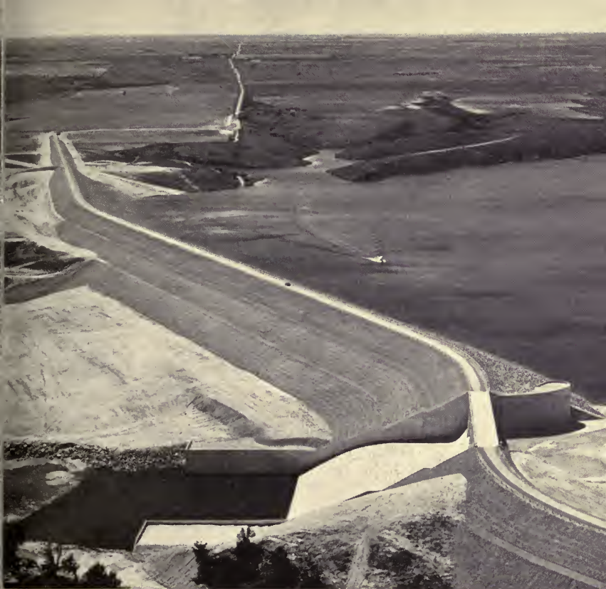
5. Medicine Creek Dam, southern Nebraska. The dam is built of rolled earth, is faced with stone, and has a concrete spillway. Lyle C. Axthelm, from BUREAU OF RECLAMATION.
