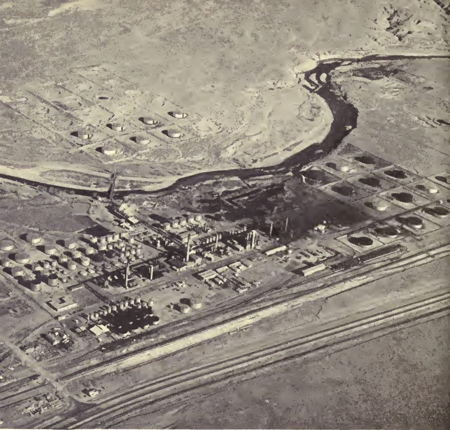
14. Large petroleum refinery on the North Platte River at Casper, Wyoming.
