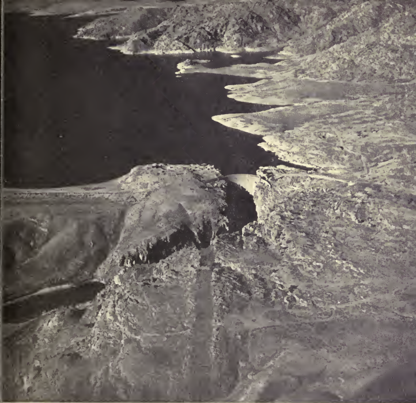
3. Pathfinder Dam on the North Platte River, Wyoming, built 1905-9. R. D. Dirmeyer, from BUREAU OF RECLAMATION.
