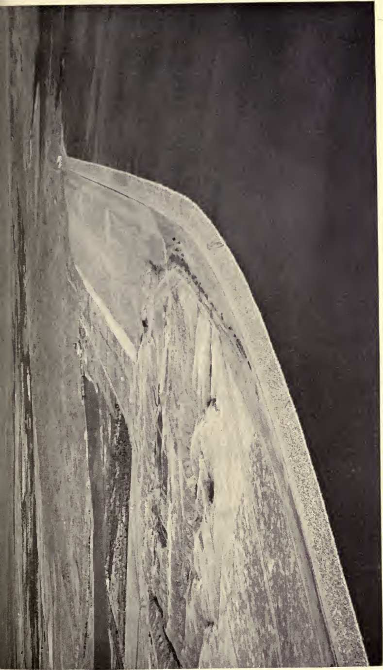
9. Fort Peck Dam, Montana. This has been the world's largest earthen barrier, four miles long. The huge reservoir ends at the rock-faced upstream dam wall.
