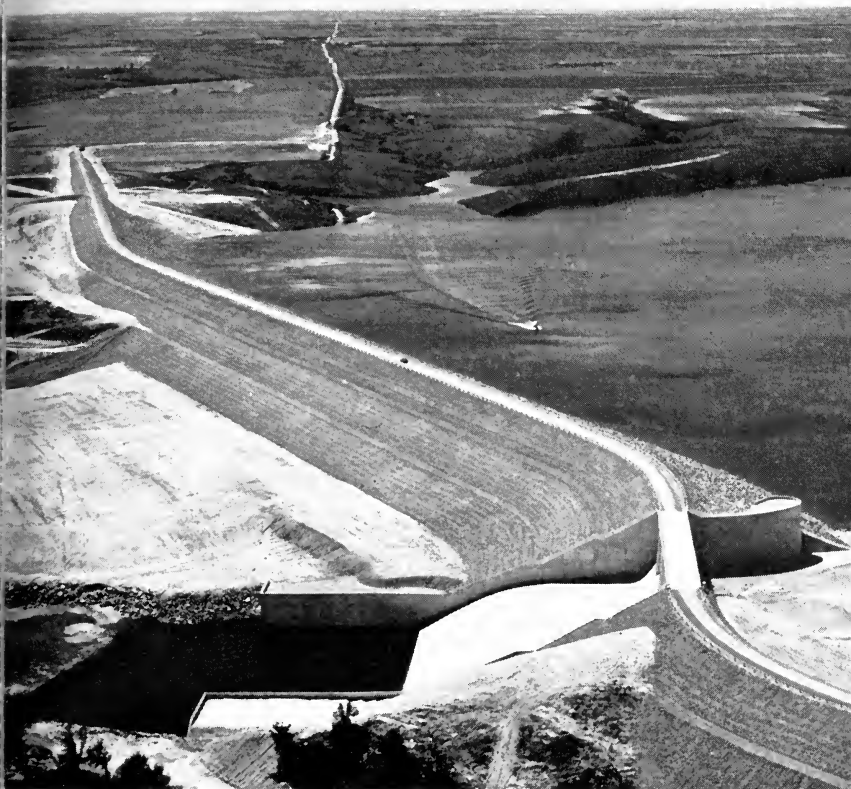
5. Medicine Creek Dam, southern Nebraska. The dam is built of rolled earth, is faced with stone, and has a concrete spillway. Lyle C. Axthelm, from BUREAU OF RECLAMATION.
