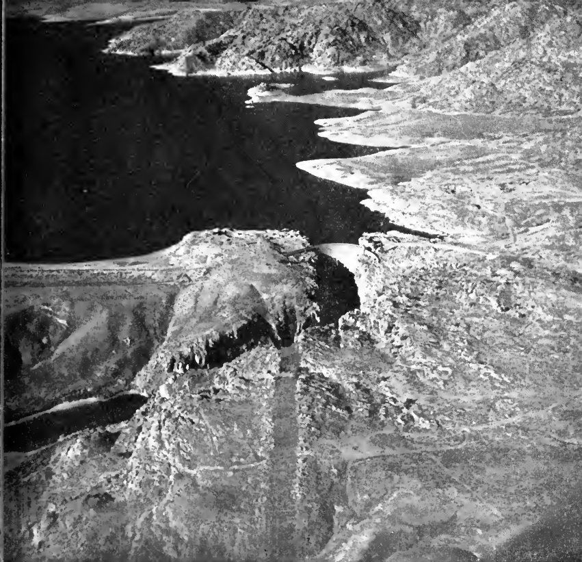
3. Pathfinder Dam on the North Platte River, Wyoming, built 1905-9. R. D. Dirmeyer, from BUREAU OF RECLAMATION.
