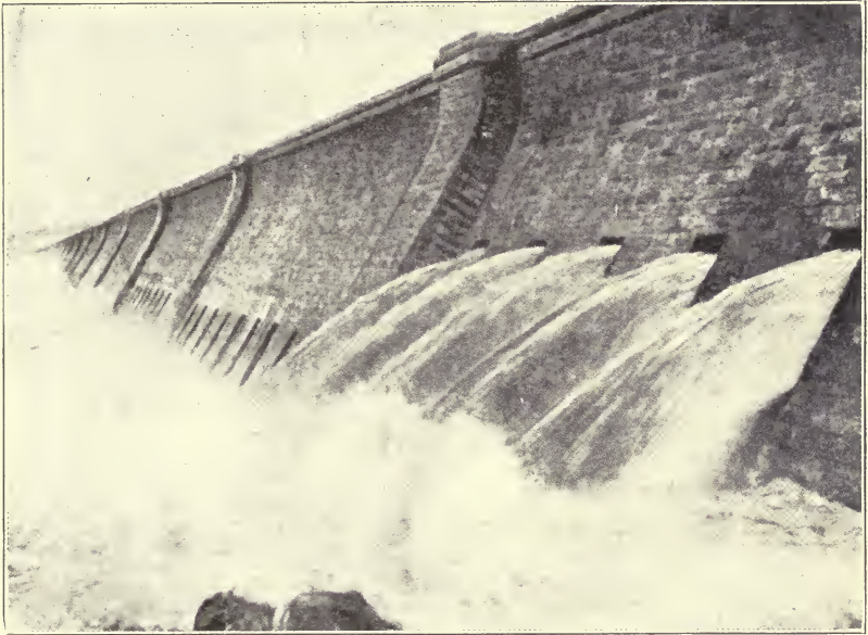
Fig. 32. View of Assuan Dam before Being Heightened with Sluices in Operation
