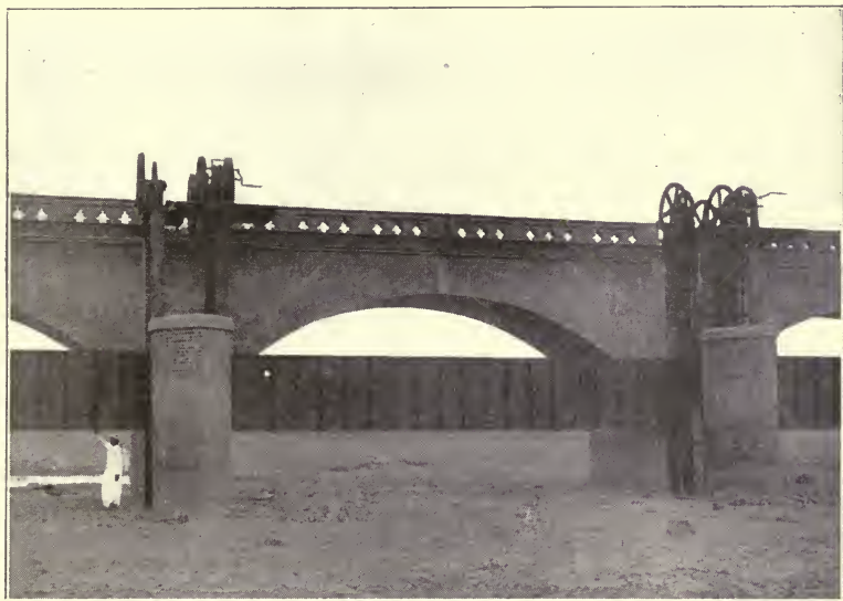
Fig. 119. View of Regulating Bridge on the Upper Coleroon River, Southern India
