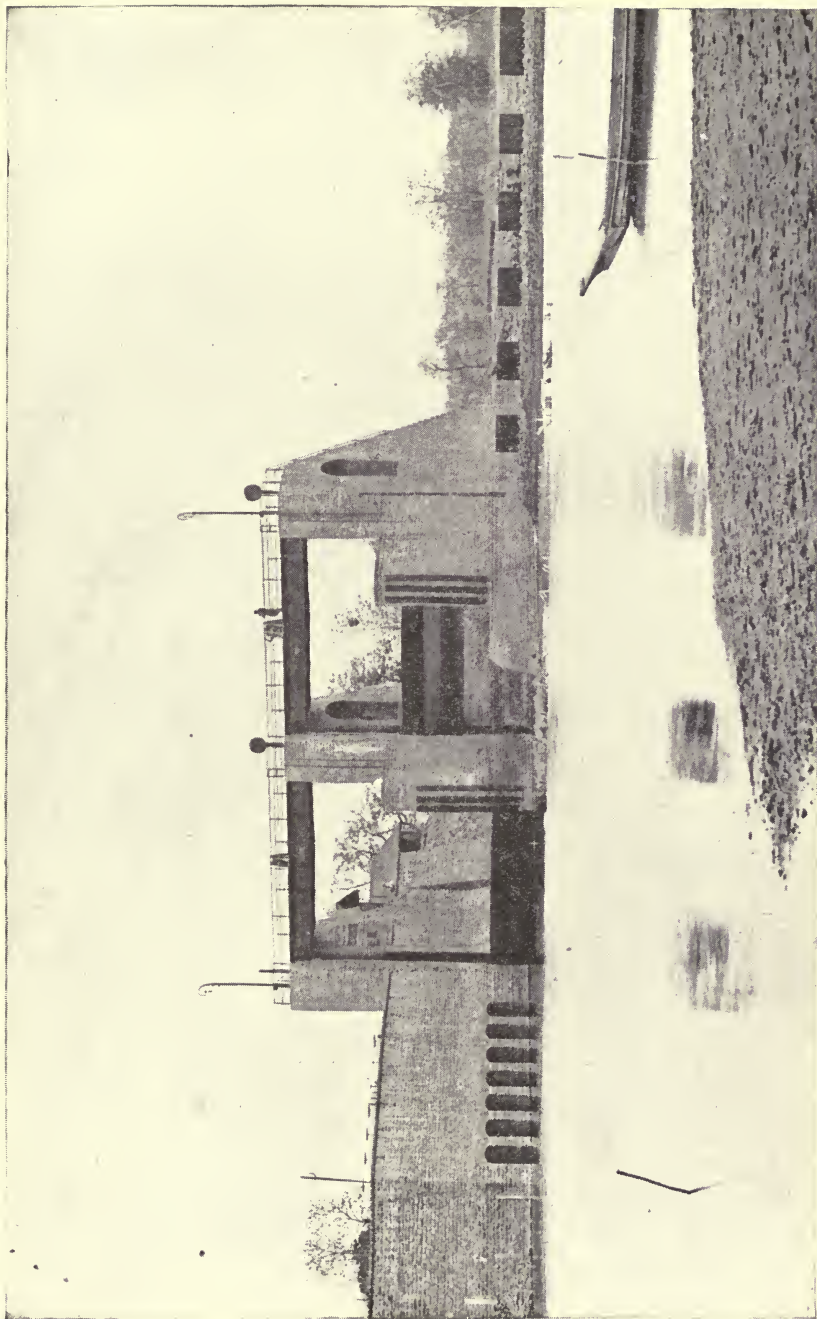
Fig. 118. Head Regulator and Undersluices of North Mon Canal in Burma, Showing Portion of Weir
