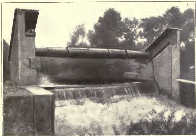
Fig. 122. View of Lauchli Automatic Dam Which Has Been for Several Years in Successful Operation in Europe
