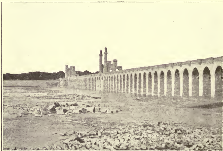
Fig. 90. View of Grand Barrage over Nile River
