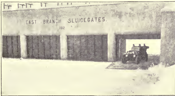
Fig. 117. Typical American Regulating Sluices in Reinforced-Concrete Weir
