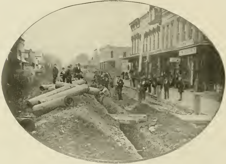
LAYING PIPES FOR DANSVILLE'S FIRST WATER WORKS
