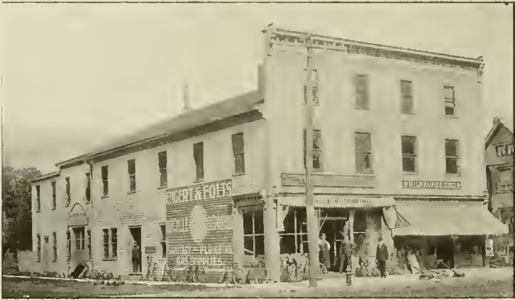
STORE AND SHOPS, ENGERT & FOLTS
