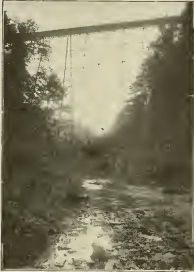
BRIDGE CROSSING STONY BROOK GLEN (COURTESY OF LACKAWANNA RAILROAD.)
