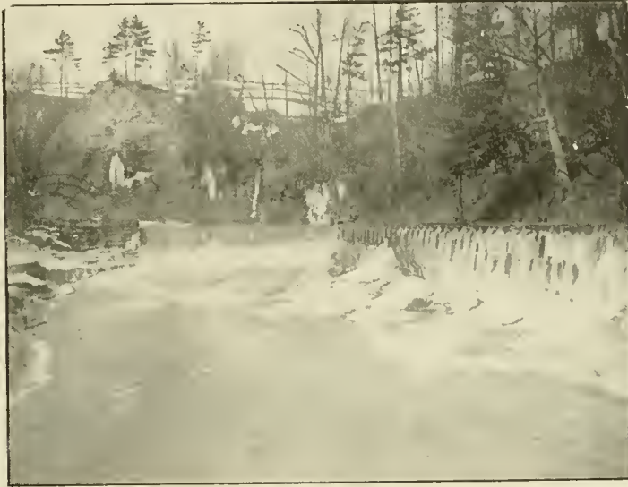
ARTMAN'S DAM AND ENTRANCE TO POAGSHOLE
