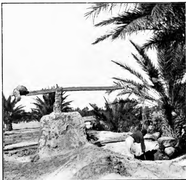
FIG. 2.—SHALLOW WELL USED TO IRRIGATE DATE PALMS AT FOUGALA, ALGERIA.
