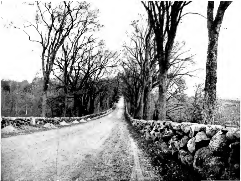
NEWBURYPORT TURNPIKE IN TOPSFIELD
