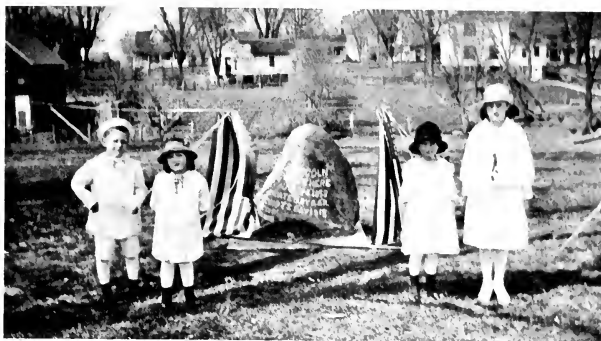
LINCOLN MEMORIAL ERECTED IN AUGUSTA, ILL.
