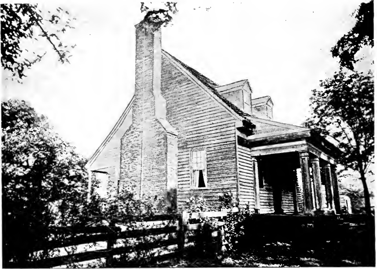
"BLOOMSBURY," HOME OF COL. JAMES TAYLOR 2D BUILT IN 1722. OLDEST HOUSE IN ORANGE COUNTY, VA.
