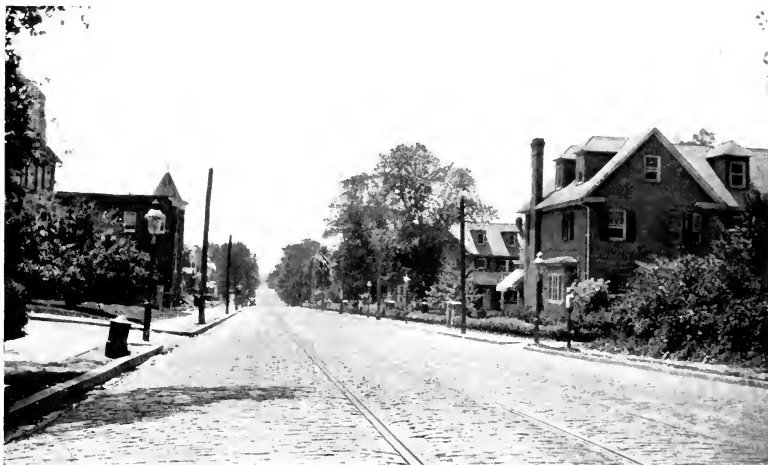
YORK ROAD, MARYLAND SCENE IN GOVANS ON THE OLD YORK TURNPIKE
