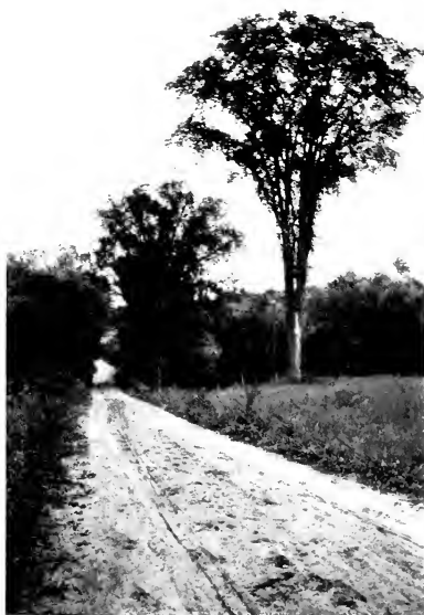
PORTSMOUTH STREET, CONCORD, N. H. ORIGINAL FIRST NEW HAMPSHIRE TURNPIKE
