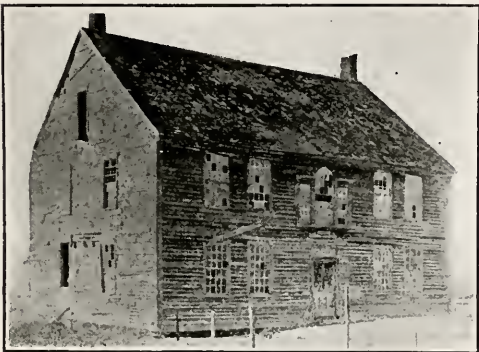
Old Harmon Tavern, built about 1770, kept by Daniel Harmon. Here Stark took breakfast on his way to Bennington.
