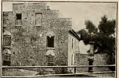
Stark Paper Mill, North Bennington, Vt. The caps over the windows and doors are made from the old mill stones used to grind corn night and day to feed Stark's army.
