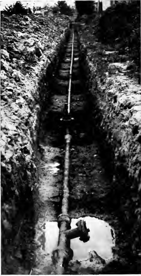
FIRST WATER PIPES LAID—TILLOLOY, APRIL-MAY, 1921
