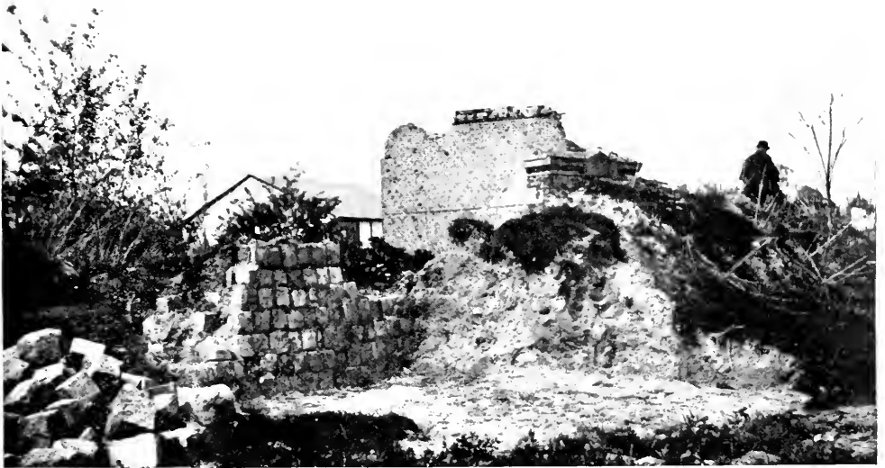
SITE CHOSEN FOR FOUNTAIN. THE PILE OF BRICKS AND THE WALL WERE CLEARED AWAY AND THE MUDDY ROAD WAS PAVED
