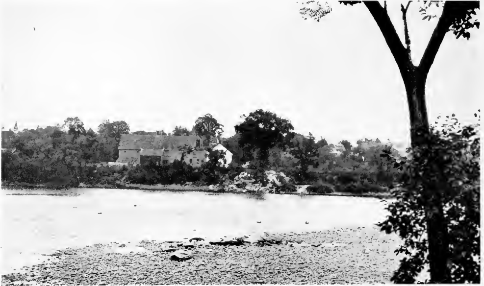
THE OLD ABUTMENTS ON THE NEW HAMPSHIRE SIDE
