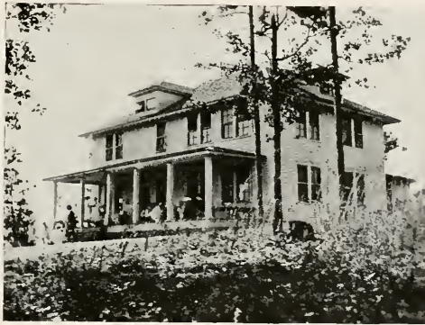
MAIN BUILDING CONTAINING SCHOOL ROOM, LIVING ROOMS AND DORMITORIES
