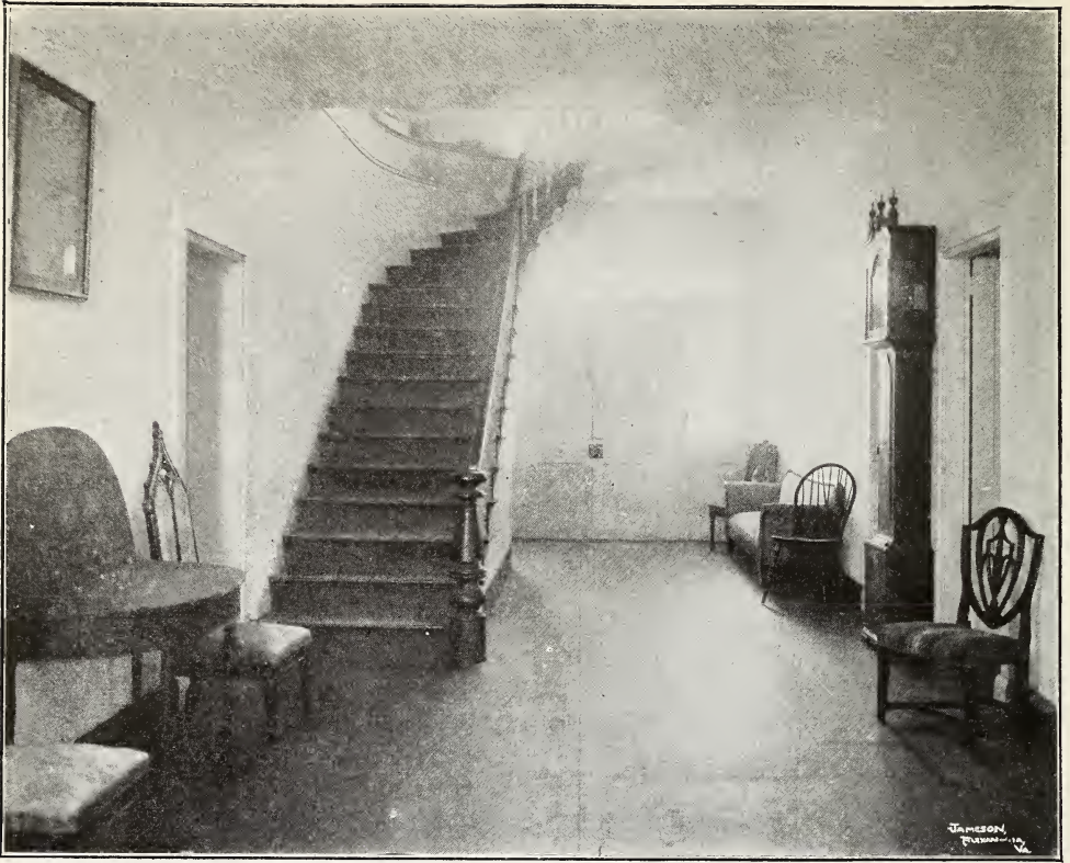
The Old Stairway and the Hall
