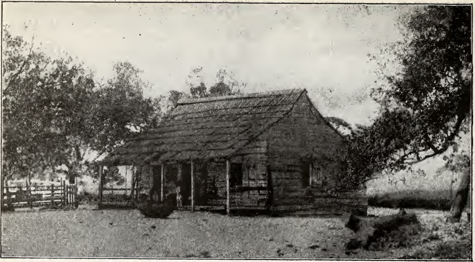
The Old Cuevas' Homestead on Cat Island, Built in 1812. The "Baton" Window with Its Iron Bolt Is Typical of the Spanish-French Mode of Building of That Period. The inevitable "Sugar Kettle" Is Seen. In These Days Every Householder Raised His Own Sugar-cane and Did His Own Boiling. This Was Known as "Open-kettle" Sugar and Molasses
