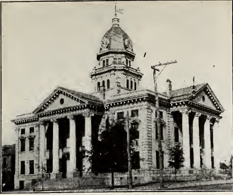
Crisp County, Ga., Court House
