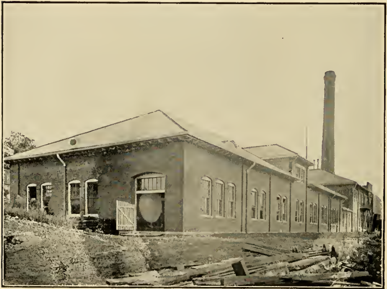
WATER WORKS. — Pumping Station No. 1.
