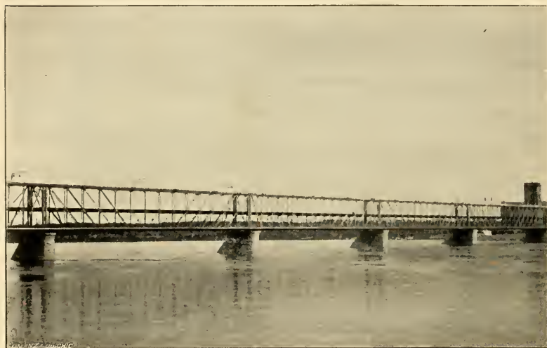
GOVERNMENT BRIDGE. — Over Mississippi.
