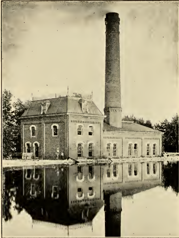
PUMPING STATION No. 2.—Reservoir.
