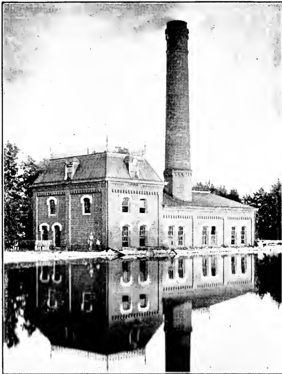
PUMPING STATION No. 2. — Reservoir.
