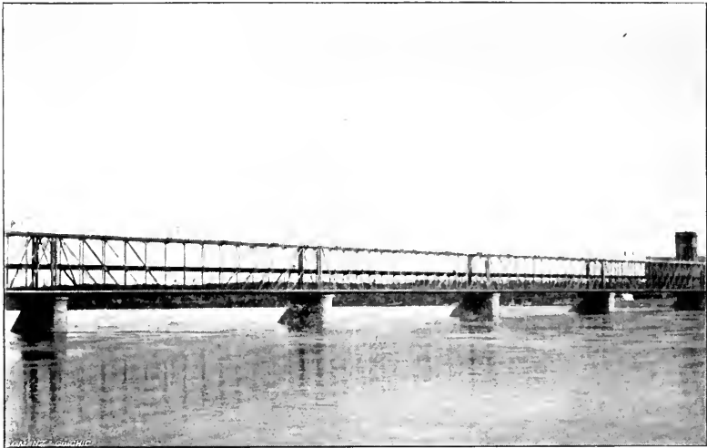
GOVERNMENT BRIDGE. Over Mississippi.
