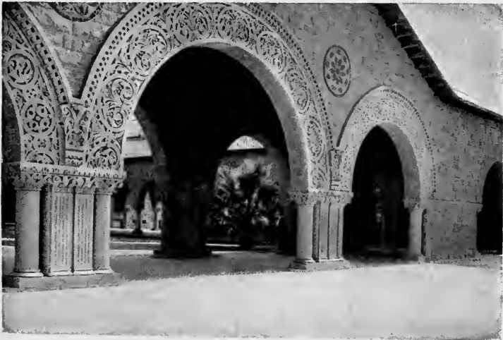
LOOKING THROUGH TRIPLE ARCH, INNER COURT, INTO MEMORIAL COURT
