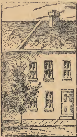
BROCK STREET SCHOOL, TORONTO.
