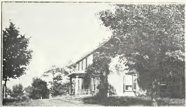
Van Bergen House, Leeds. H. F. Vedder, Owner.
