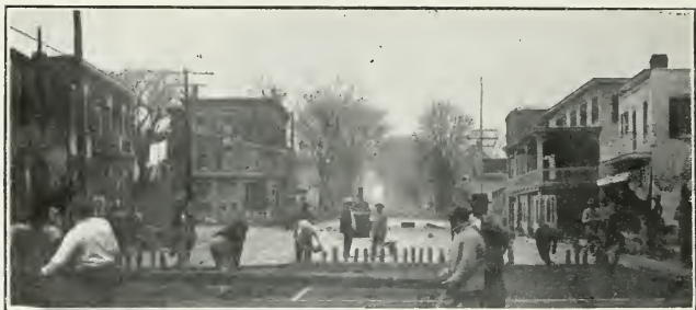
Laying Brick Pavement, West Bridge Street.
