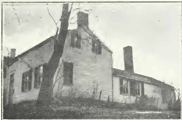
The Oldest House on William Street, 1798.
