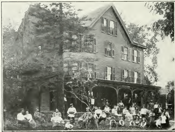
Little Falls House, South Cairo, Destroyed by Fire 1914.
