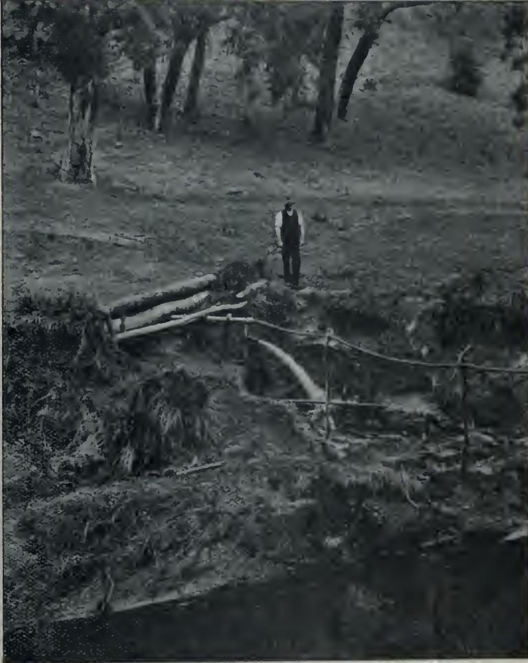
Another View of the Spring. (The Pipe shown is fitted to the Bore ready for Canning).
