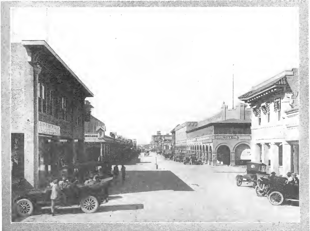
Looking Down One of El Centro's Busy Business Streets.
