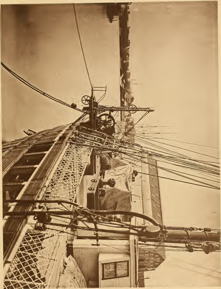
THE SIDE SOUNDING MACHINE IN POSITION. RUN OUT FOR WORK.
