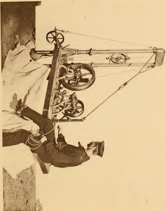
THE SISBEE SOUNDING MACHINE RIGGED FOR PAYING OUT.
