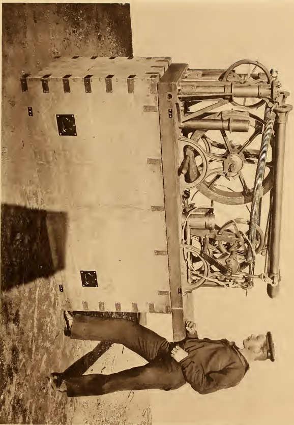
THE SIBSBE SOUNDING MACHINE FOLDED FOR TRANSPORTATION.
