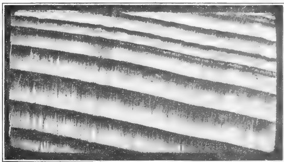
FIG. 5.—Cross section from an unfinished elevator beam, showing a lightning ring in Sitka spruce. The row of resin ducts extending entirely across the section can be seen in the summer wood of the fifth annual ring from the bottom. The defect ran the entire length of the beam.
