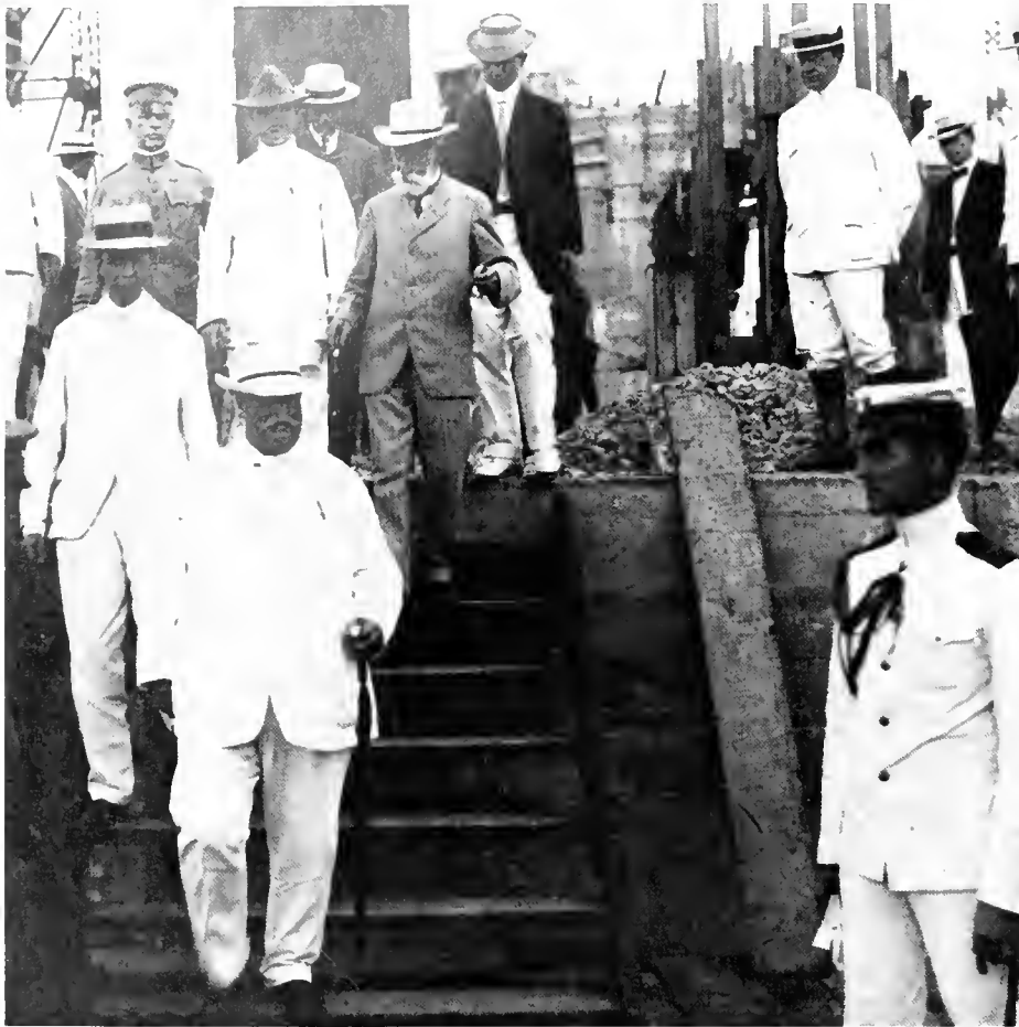
As President-elect, William Howard Taft visited Panama in 1909 to inspect construction of the canal.
