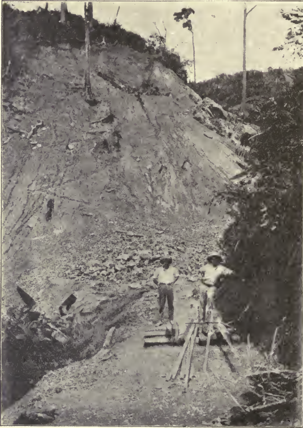
FIG. 273.—Open-cut of the Rahman Tin Co., near Intan, Perak, showing wide shattered lode in slate.
