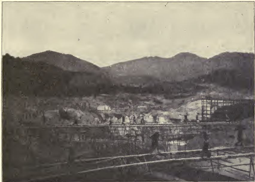
FIG. 274.—Open-pit workings at Jelapang, near Ipoh, Perak. Gravel-deposit upon limestone. Granite hills in the distance. Wolff.
