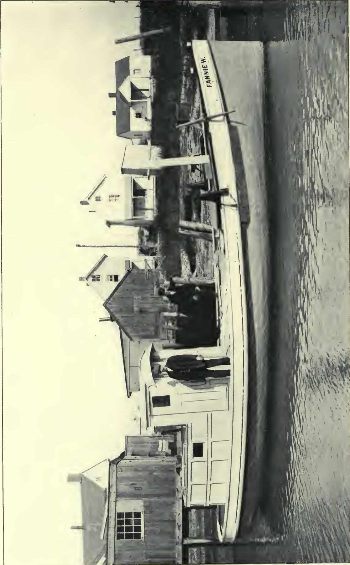
OYSTER DREDGE FANNIE W., OWNED BY SPRAGUE & DOUGHERTY, OYSTER PACKERS OF INWOOD, L. I., N. Y. 35 feet O. A. by 10 feet beam. Buffalo 2-cylinder 6 by 7½ inches bore and stroke, 13-15 horsepower. Heavy duty type. Columbian propeller 20 by 24, Style B, 350 revolutions per minute. Double ignition, separate plugs; starts on Delco batteries with Bosch magneto. Gasoline fuel; about 1½ gallons per hour. This work boat is at least 20 years old and her present power plant has been in service for more than six years and is still in excellent condition. She has a capacity of 400 bushels of oysters and when loaded makes about 8½ miles per hour.
