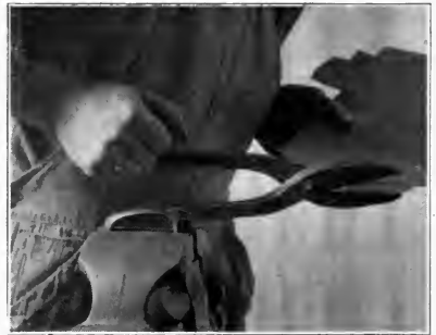
Fig. 105. Cutting copper with snips.
