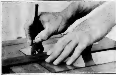
Fig. 84. Cutting glass. (Step 1.)
