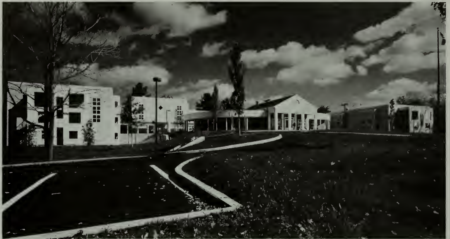
Michael R. Koury Terrace Torrington, Connecticut Ulrich Franzen & Associates, Architects
