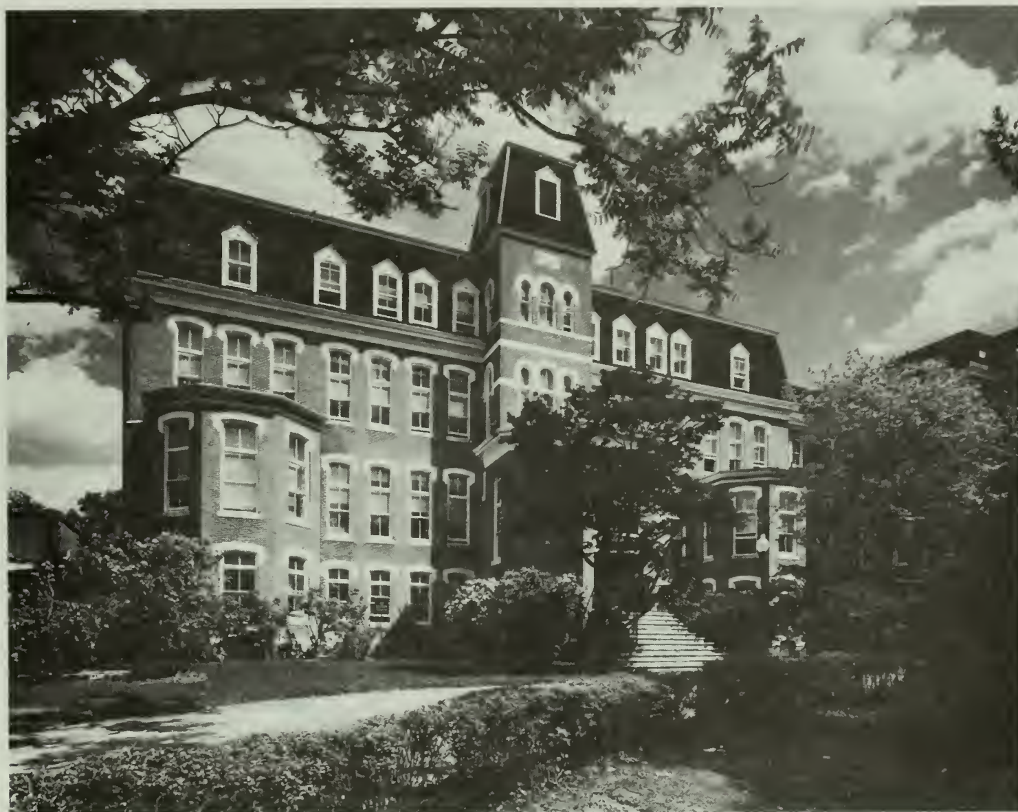
Lafayette Place Fall River, Massachusetts Boston Architectural Team, Inc. Hresko Associates, Boston Phillip Hresko, Principal David Clark, Job Captain Nick Wheeler, Photographer
