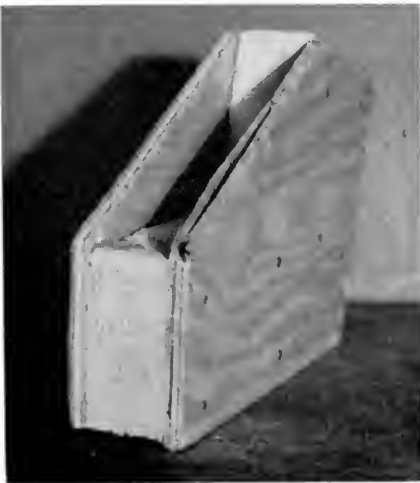
The compression edge of 3/8-inch gussets must be supported to prevent buckling failures of the type shown. (Fig. 5)
