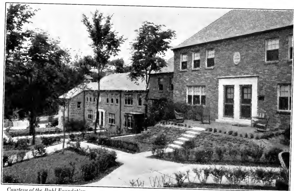
Courtesy of the Buhl Foundation.
