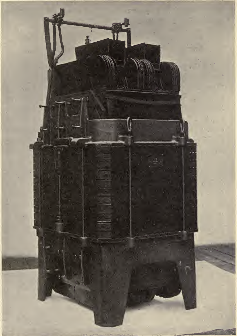
FIG. 6.—100-kva single-phase 100 000-volt shell-type transformer built by the Westinghouse Co. for the Southern Power Co.
